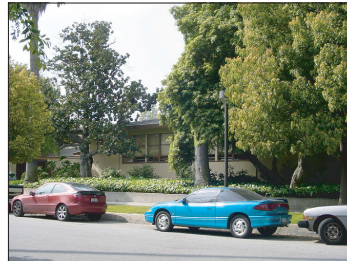
Photo 4 - Photo taken from Holliston Avenue illustrates size and scale of existing Plant Offices and Shops.
