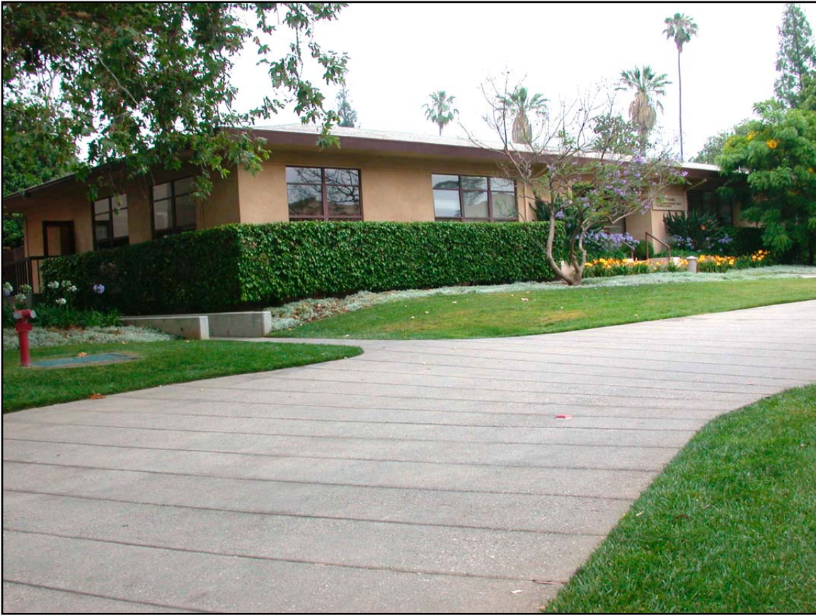
Photo 1. Physical Plant building, southern and western elevations. [16 June 2005]
