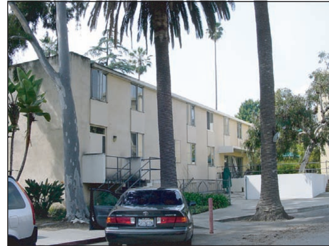
Photo 2 - View of northern facade of Marks House from rear parking lot.
