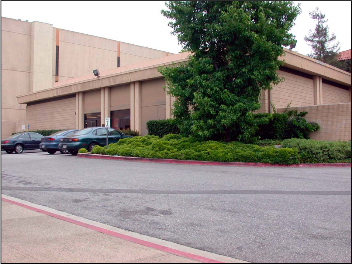
Photo 5. Mead Labs building, western and southern elevations. [16 June 2005]
