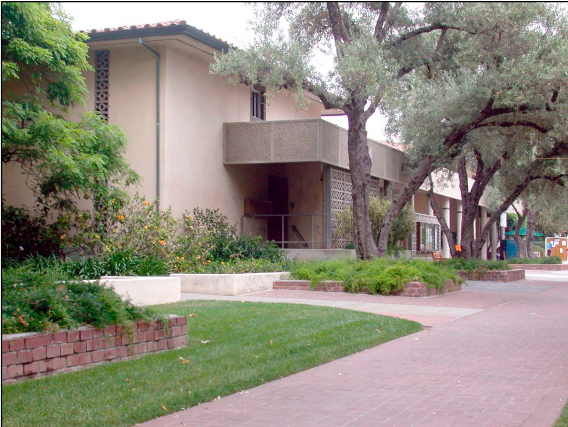
Photo 4. North Undergraduate Houses, southern and western elevations. [16 June 2005]
