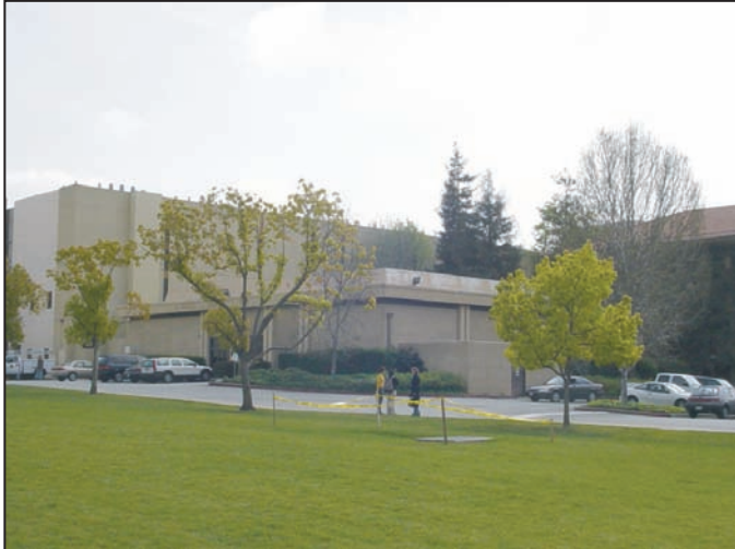
Photo 3 - View of Mead Laboratory from Wilson Avenue. Photo demonstrates disparity between the size and scale of Mead and surrounding buildings.
