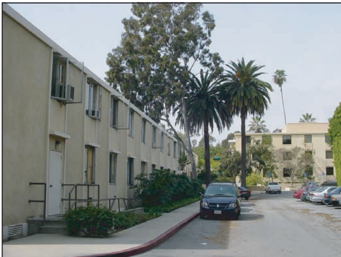
Photo 3 - Photo of northern facade of both Braun and Marks Houses showing difference in height and scale as compared with neighboring Mosher-Jorgensen House.
