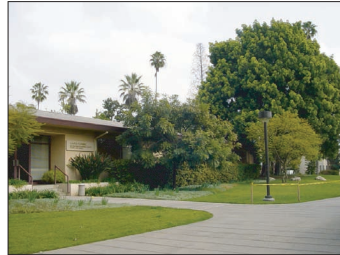
Photo 2 - Photo of Physical Plant Shops illustrates existing setbacks, landscaping, and foreground views as seen from Holliston Avenue.
