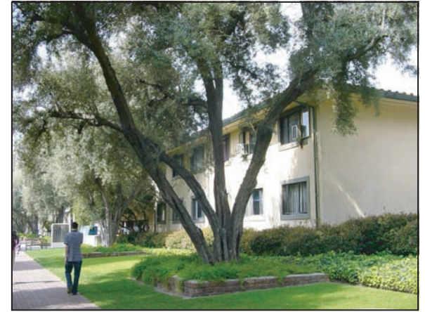
Photo 3 - View of exterior of the Lloyd House (facing west) from the open space corridor "Olive Walk."
