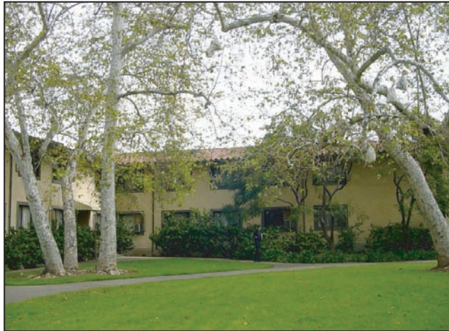
Photo 4 - View of exterior of the Page House (facing east) from unstructured open space west of North Undergraduate Houses and "Olive Walk."
